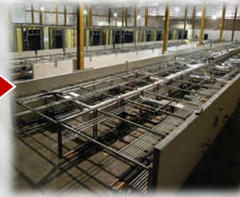
Racks Installed in Corridor
