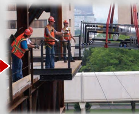
Crane Lifts Racks to Floor
