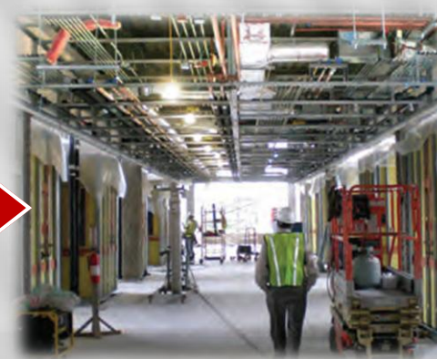
Racks Installed in Corridor
